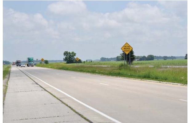
Hwy 14, facing east
