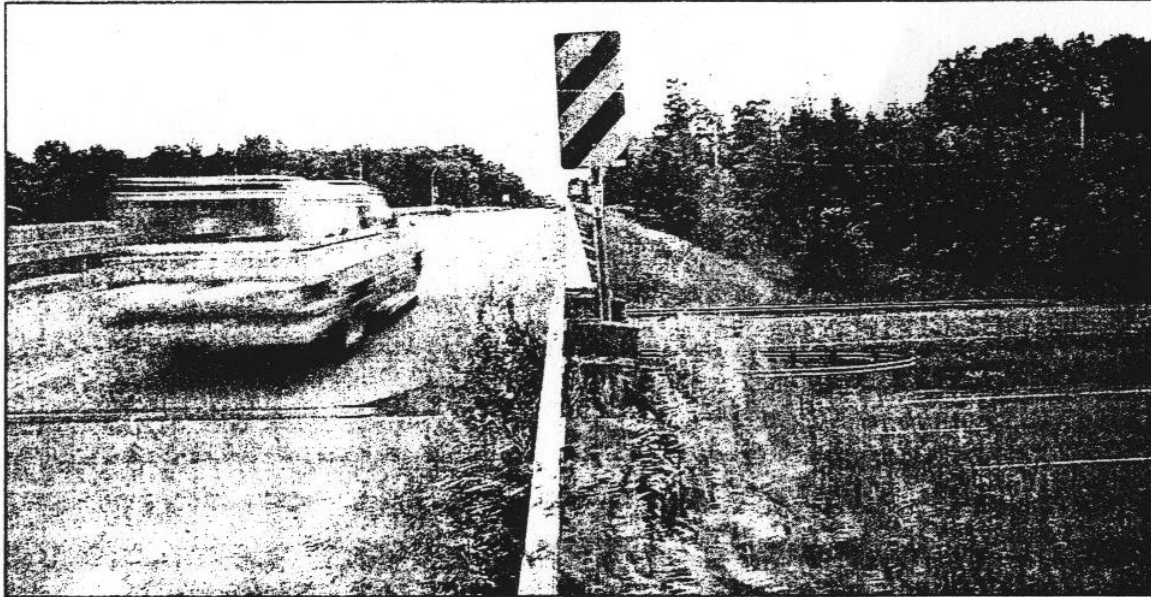
A car drives past on the Highway 45 bridge over Highway 14.
